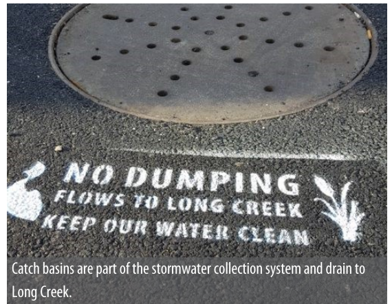
Cover all utility and catch basin infrastructure so sealant does not enter.
